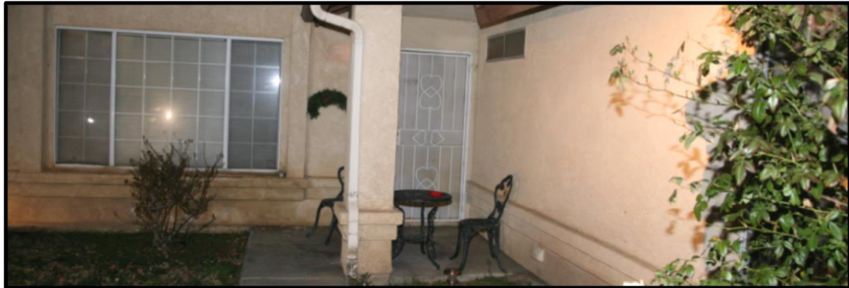
Figure 2: Photograph depicting pillar near the front door.
