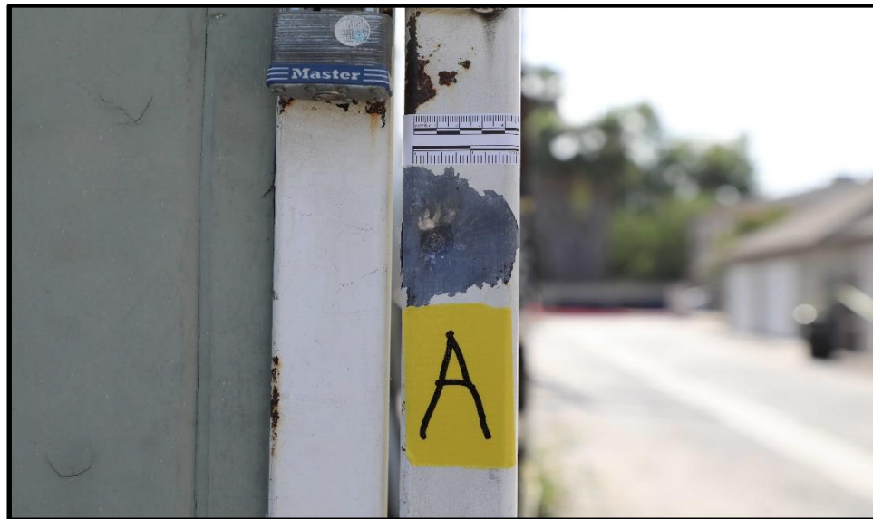
Bullet impact on the metal gate.
