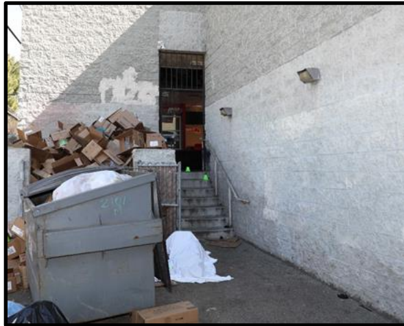
Photograph depicting steps from the trash dumpster area to the adjacent cannabis dispensary.
