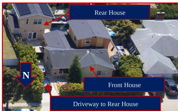
Figure 1: Photograph Depicting the Front and Rear Houses on the Flag Lot
