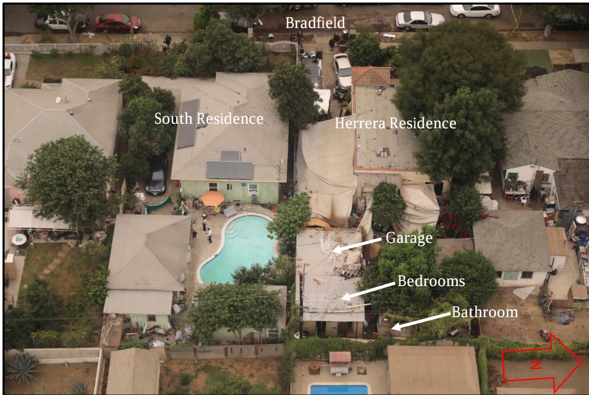
Figure 2: Aerial view of the Herrera and south residences, viewed from the east
