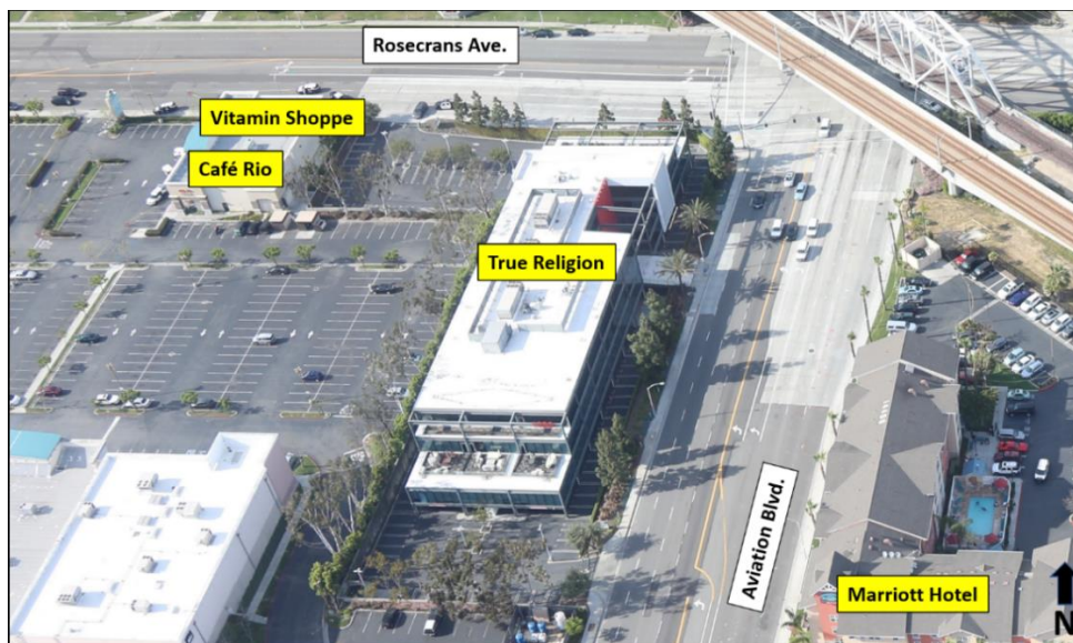
Figure 1 – Aerial photograph depicting the area of Rosecrans Avenue and Aviation Boulevard. Relevant locations are labeled in yellow.
