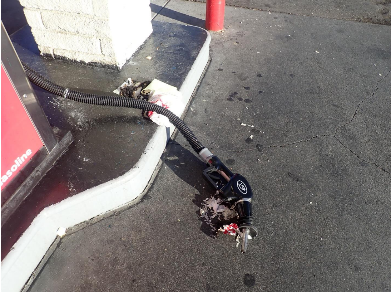
Photograph 1 - Photo of pump #1 nozzle and burnt debris.
