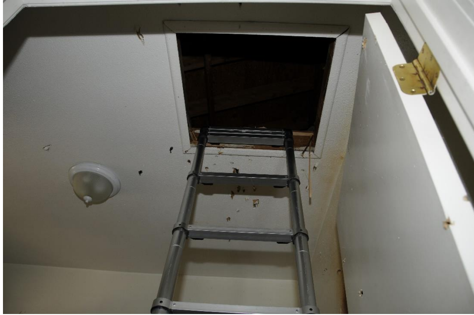
Photo of the Ladder Leading to the Attic Access Hole
