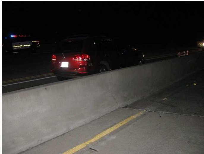
Center Divider Wall of Interstate 210 Highway
