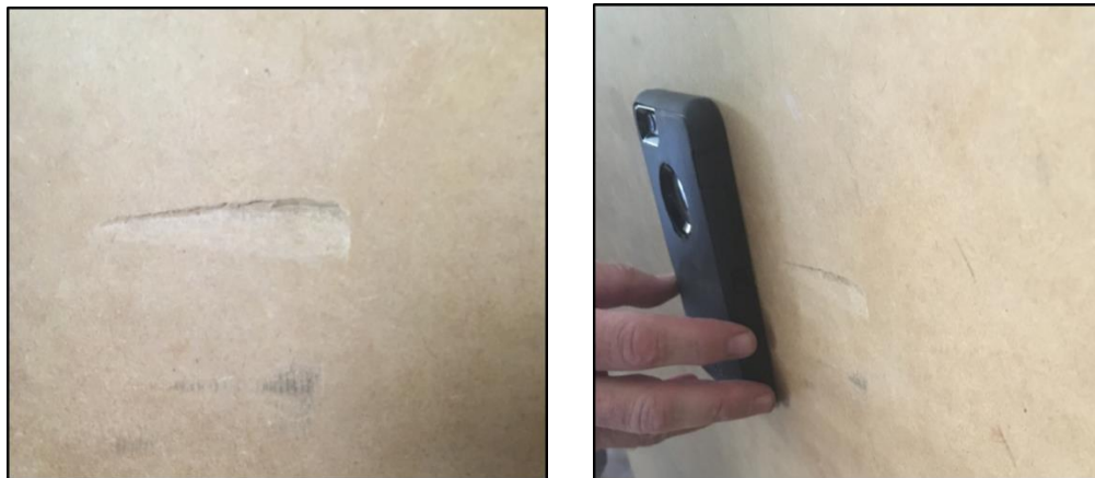
Figures 4 & 5 – Photographs of the strike mark damage located on the garage door.
