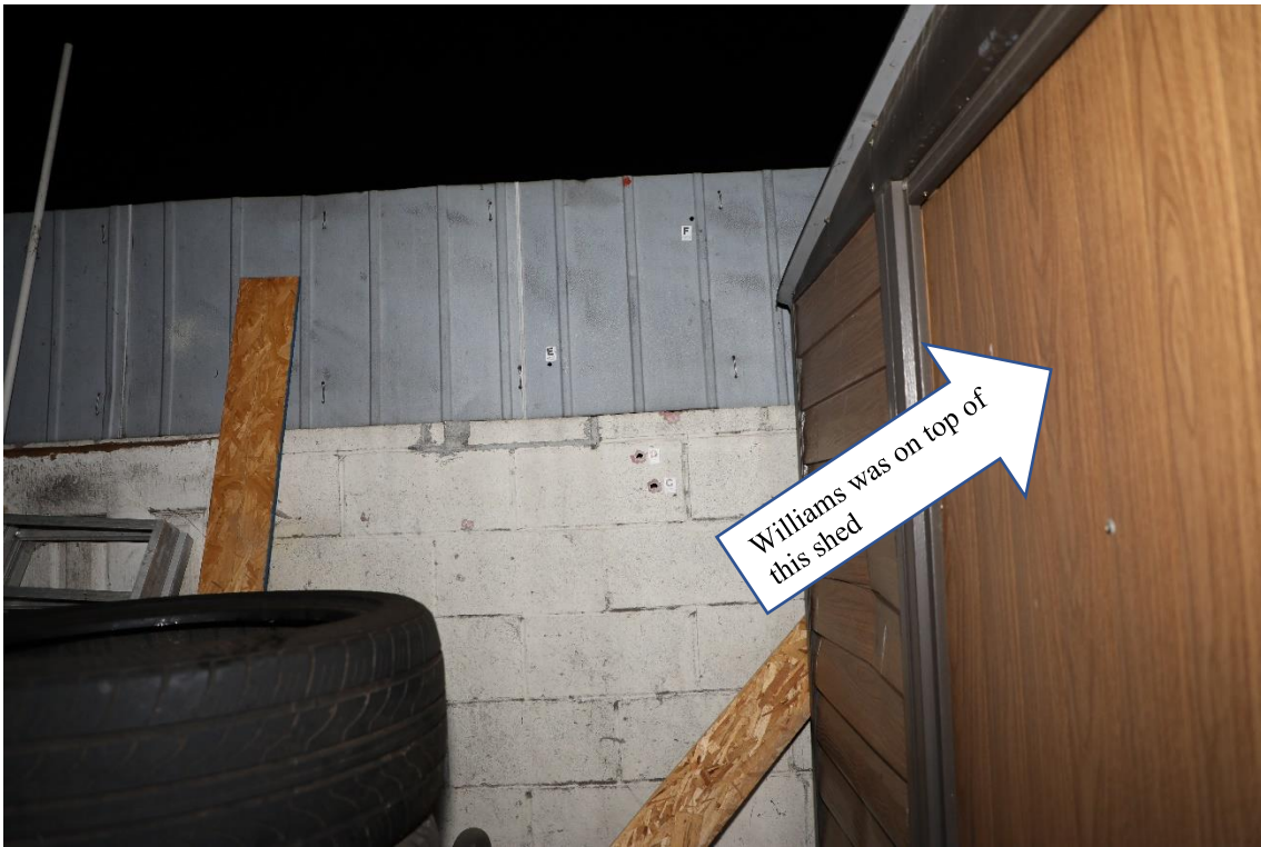
Photo depicting four bullet holes (marked C, D, E, and F) in the wall next to the shed.
